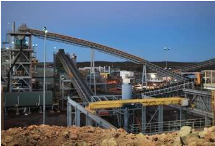
Windimurra Vanadium Project © Atlantic Ltd.
